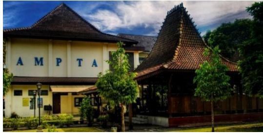
Picture 4.1 STP AMPTA Yogyakarta Building Source: Field Observation, 2023
