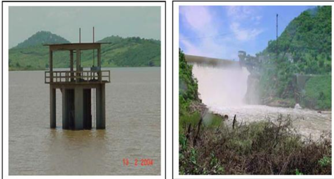
Figure 2. Water intake for the Coremas reservoir and Bleeder for Mãe D'Água reservoir. Source: Lima (2004).
